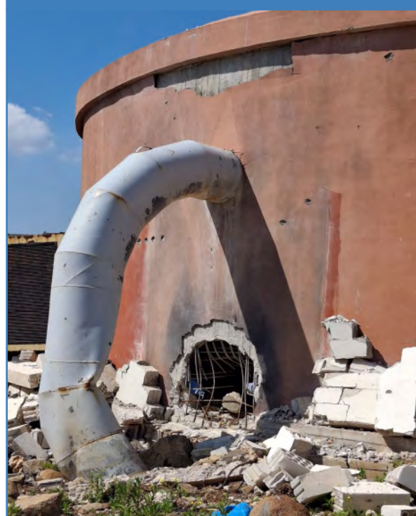
Figure 4: Photo showing damage to the water tank at the Maisat water pumping station
