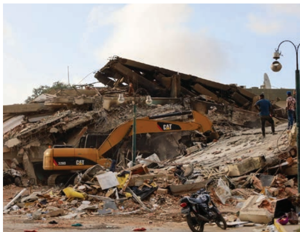
Venezuela, Collapsed buildings following the earthquake, 2026. © Elisamuel Devis Fermin ADRA
