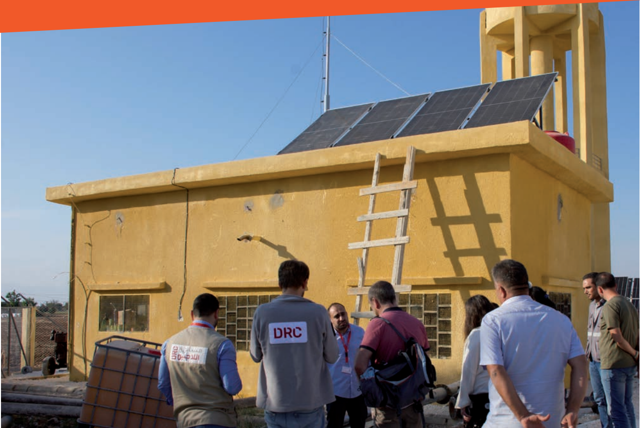
Syria: An ECHO funded, DRC community programme to rehabilitate a solar-powered borehole, bringing water to 6000 community members © DRC, 2025
