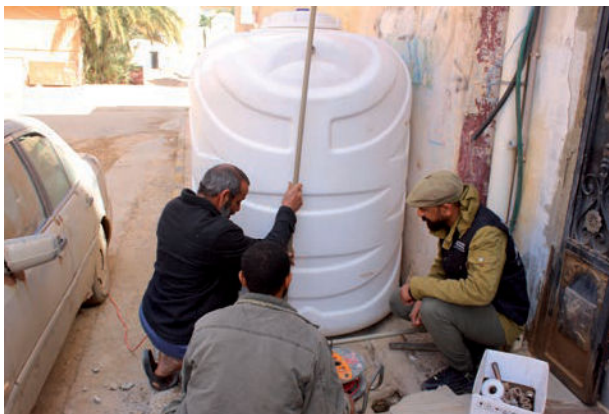
IMC staff members install the water tank near Ahmed’s house in February 2024.
