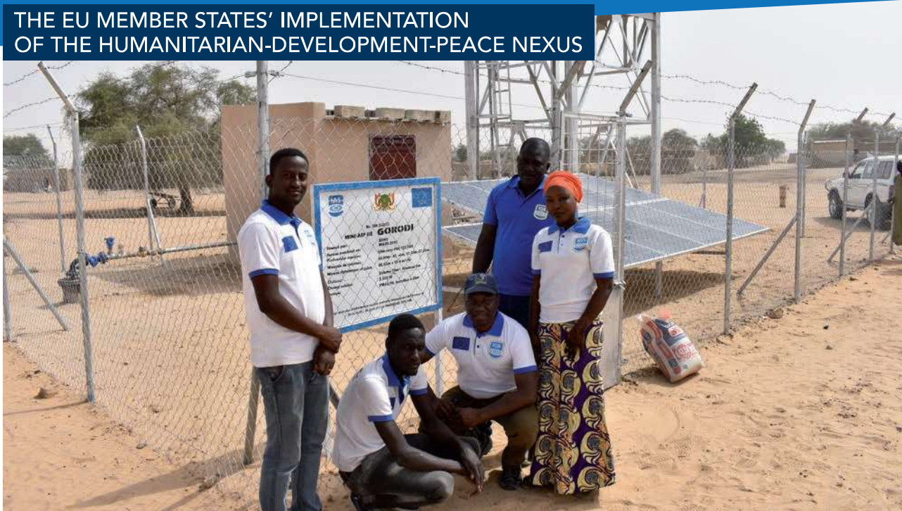
Team at a Completed Water Yard - ©: Paul Hayes (IAS Niger)
